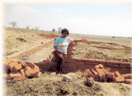
3rd Classroom Block Foundation
