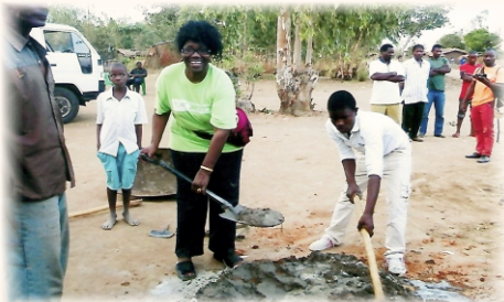
Laying the Foundation of the School
