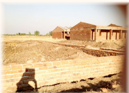
1st & 2nd Classroom Block Standing
