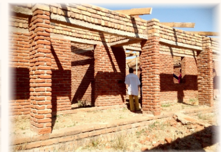
Progress on 3rd Classroom Block
