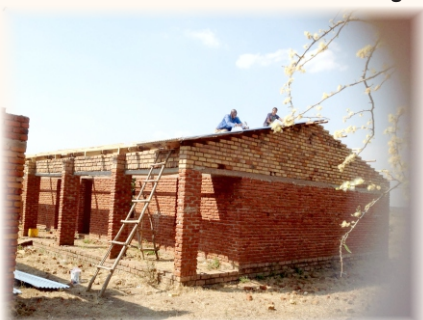
Roofing work begins
