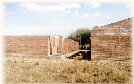
2nd Classroom Block coming Up
